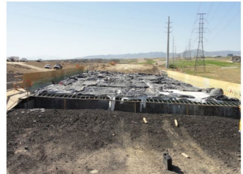
Covered bridge deck during curing.
