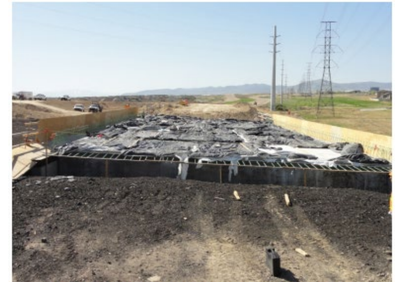
Covered bridge deck during curing.
