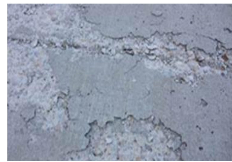
Freeze-Induced Damage in Concrete Coupal, J. (2015, January 22). Practical advice for pouring concrete walls in cold weather – Boston, MA, A-1 Foundation Crack Repair, Inc.
