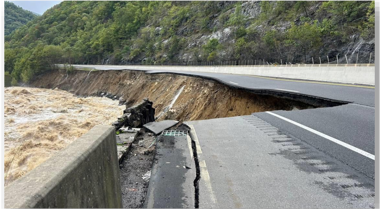
Several lanes of I-40 in N.C. near the Tennessee line washed out and collapsed during catastrophic flooding from Helene. The North Carolina Department of Transportation said I-40 was closed in multiple locations between Asheville and eastern Tennessee due to washouts and debris. NC DOT
