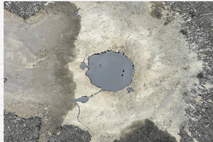
Hole filled with epoxy
