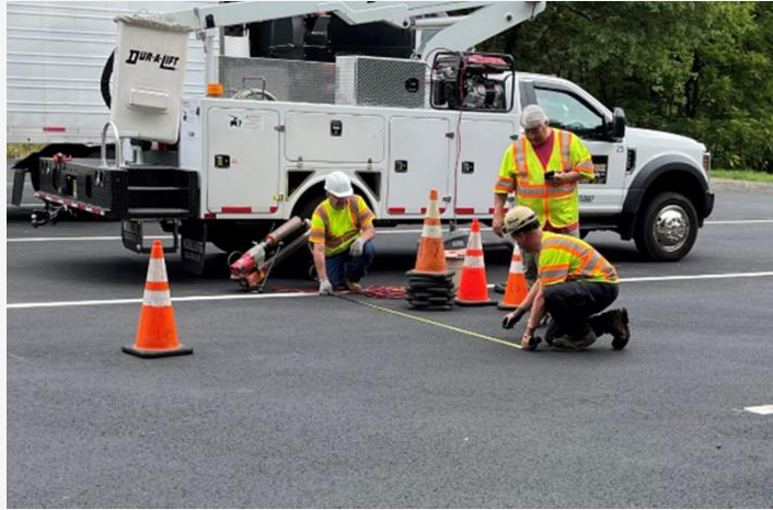
Measuring the position of a sensor hole
