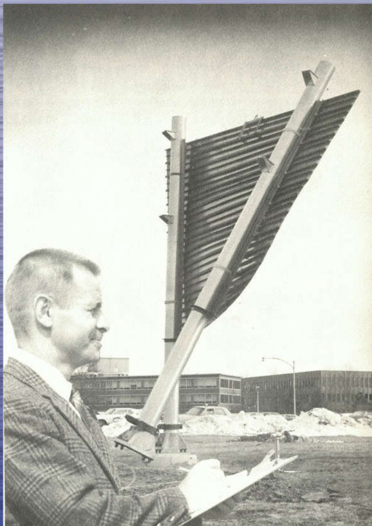
Engineer Richard A. Strizki of the New Jersey Department of Transportation makes notes on the successful L.C.B.C. Breakaway Device test.
