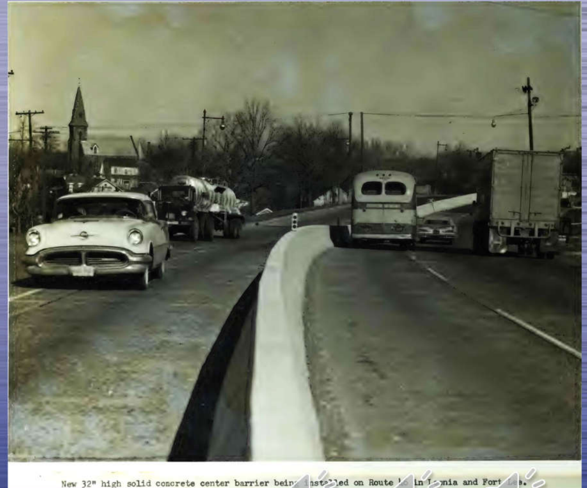
New 32" high solid concrete center barrier being installed on Route 1 in Fort Lee.
