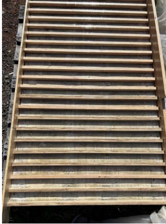
Figure 16. Formwork for Plain Slab
