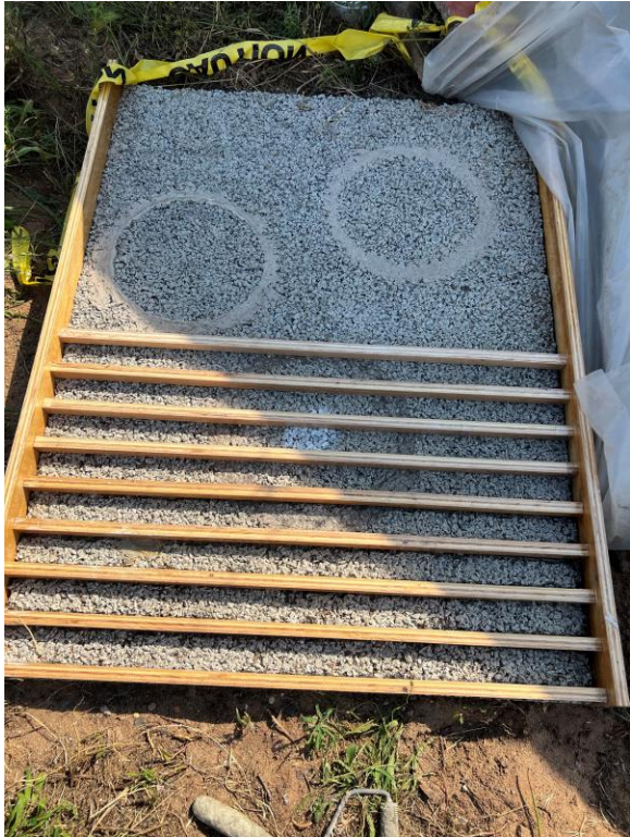
Figure 15. Formwork for porous slab
