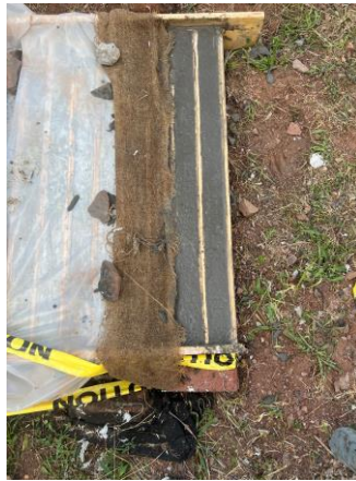
Figure 19. RS samples curing with burlap
