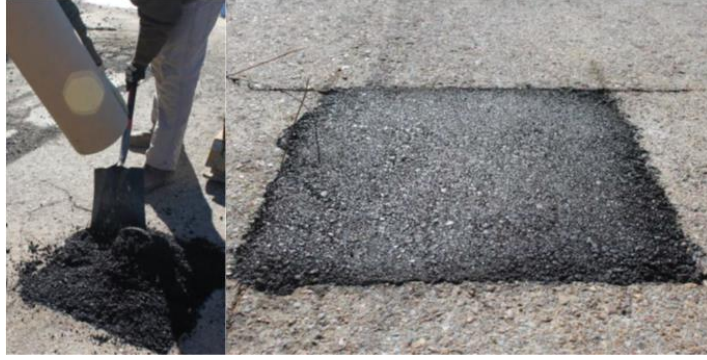
Figure 23. Field repair of pothole using induction heating (59)
