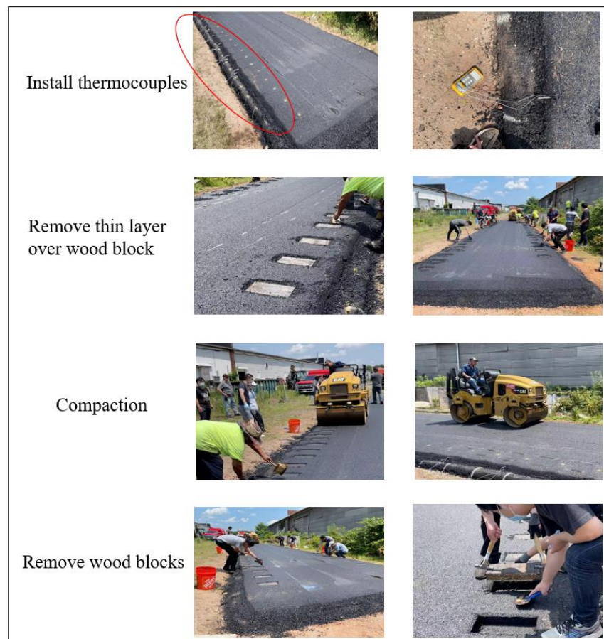
Figure 35. Second layer construction
