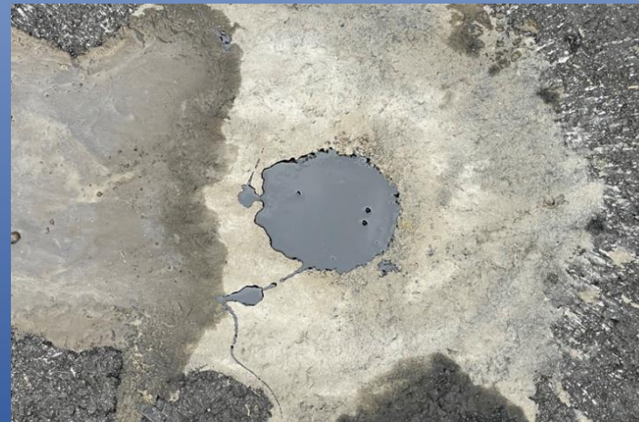
Hole filled with epoxy
