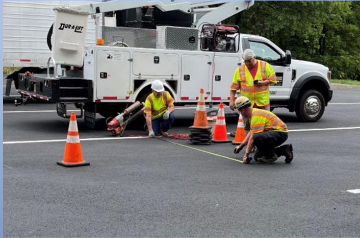
Measuring the position of a sensor hole
