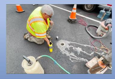
Measuring the position of a sensor hole
