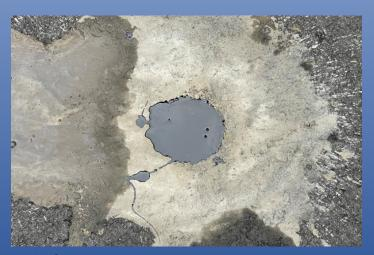
Hole filled with epoxy
