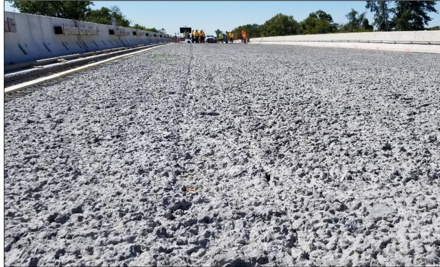
Hydrodemolished Surface – Typical
