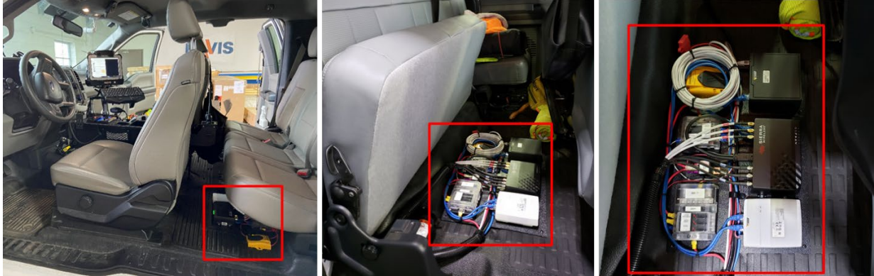
Figure 12. The camera main unit (Axis F41), PoE injector, cellular LTE modem, and the power distribution unit installed under the back seat of an IMRT (F-250) and SSP (F-350) trucks (Source: NJIT)
