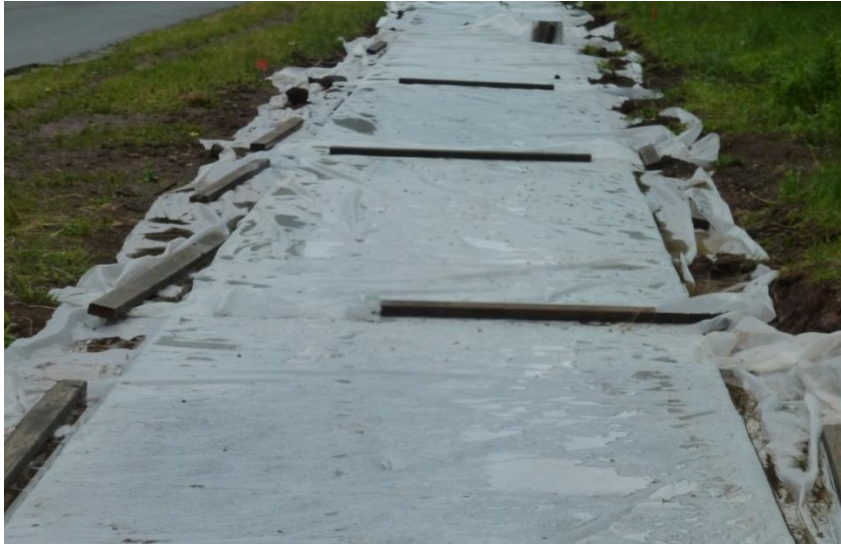
Figure 20. Curing of porous sidewalk using polyethylene sheets
