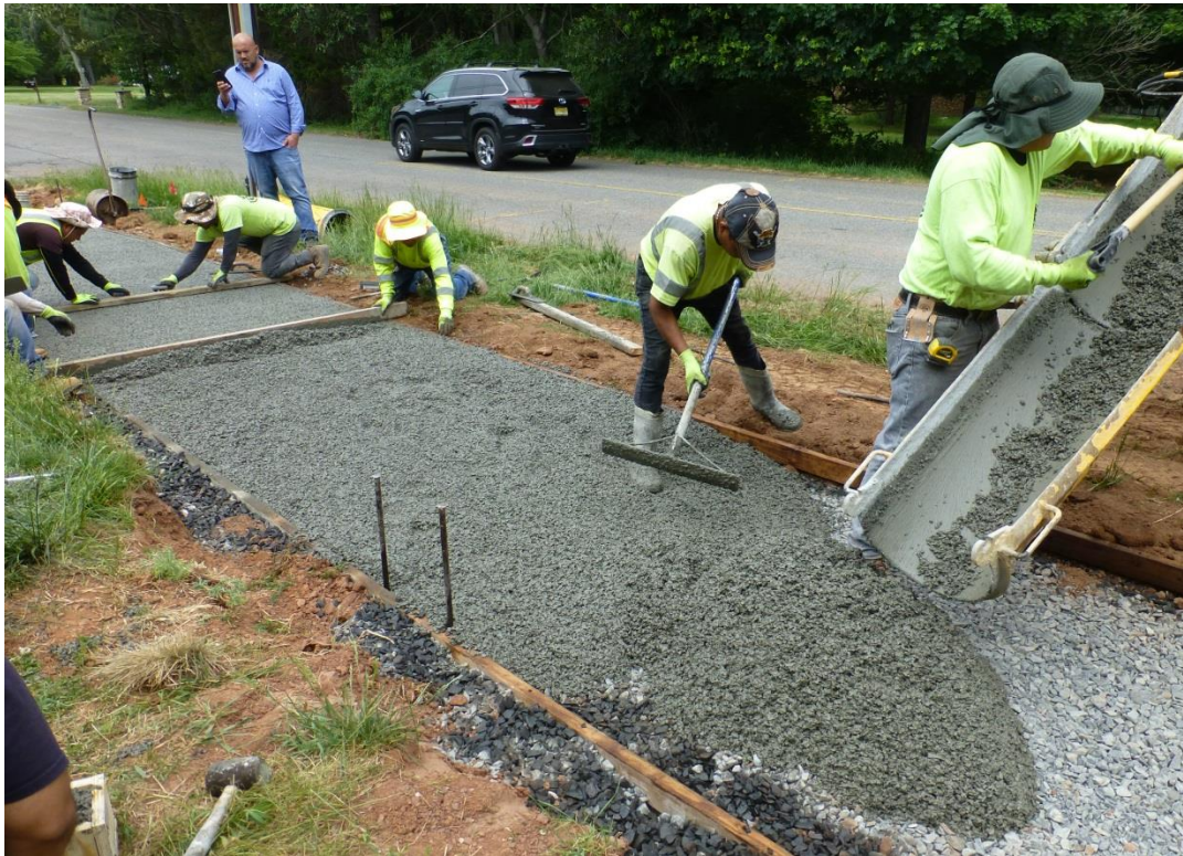
Figure 17. Porous concrete placement
