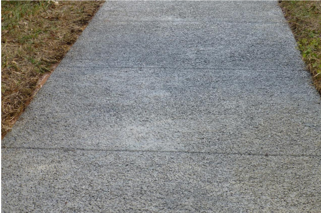
Figure 31. Finished porous concrete sidewalk after pressure washing
