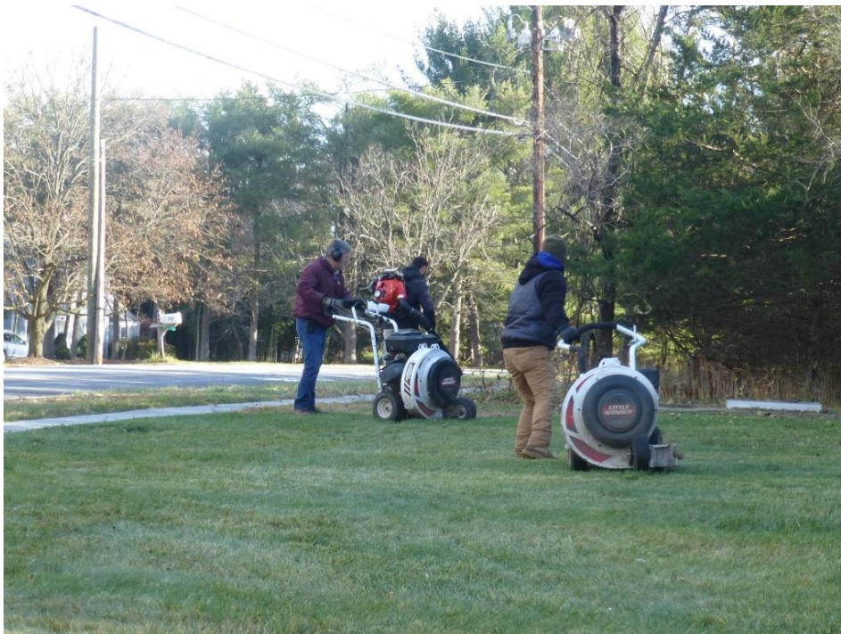
Figure 27. Cleaning the porous sidewalk using 'walk behind' vacuuming machines.
