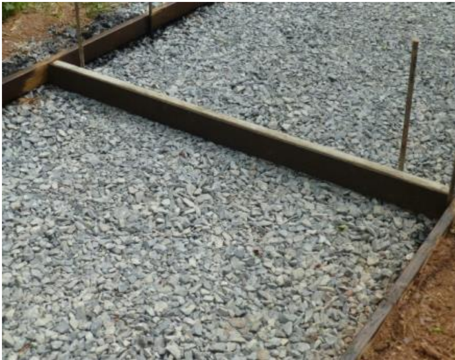
Figure 15. Location of expansion joint (every 15 ft)
