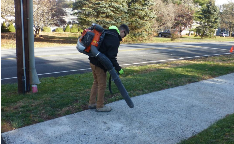
Figure 26. Cleaning the porous sidewalk using handheld air blower
