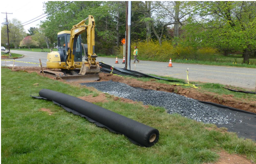
Figure 14. Placement of aggregate layer (storage layer)
