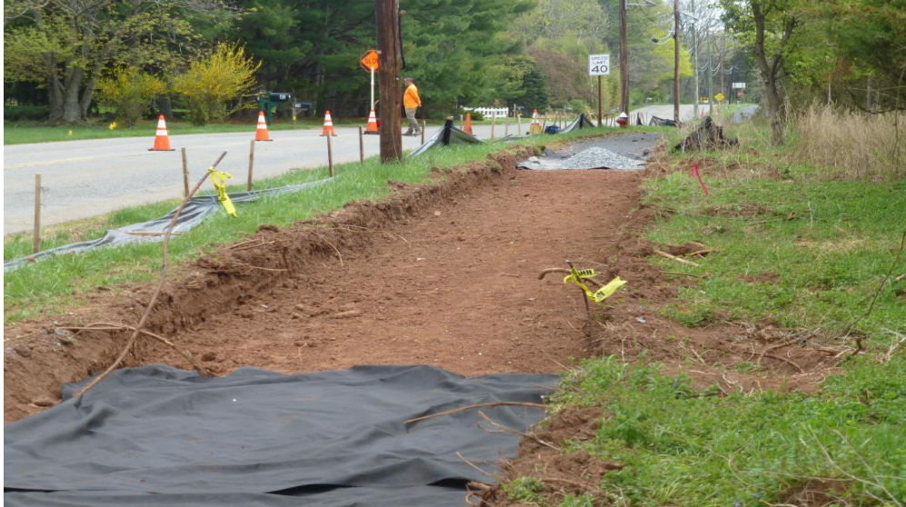
Figure 13. Excavation and placement of geotextile membrane
