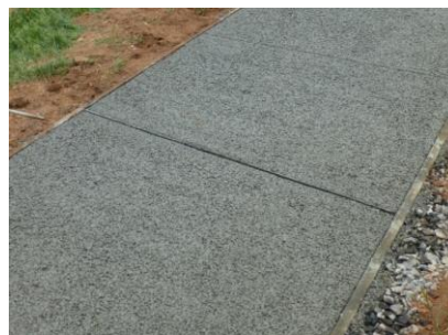
Finished porous concrete surface
