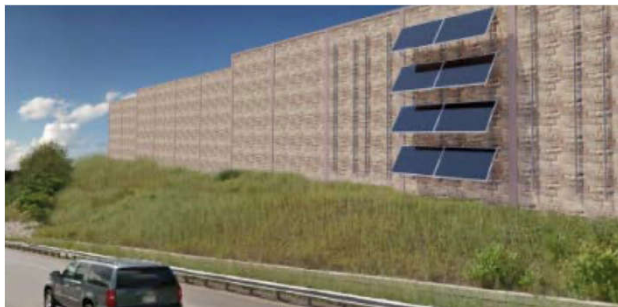
Fig 1: Visualization of proposed PVNB on existing noise barrier in Massachusetts from Massachusetts DOT
