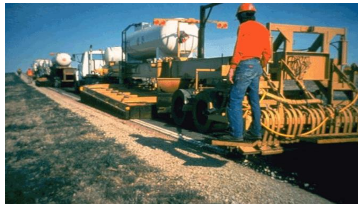
Fig. 1. Hot in-place recycling
