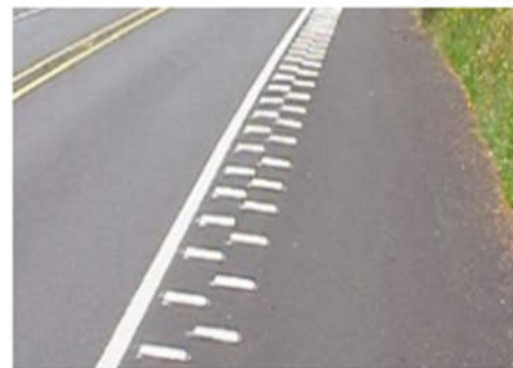
Raised Rumble Strips
