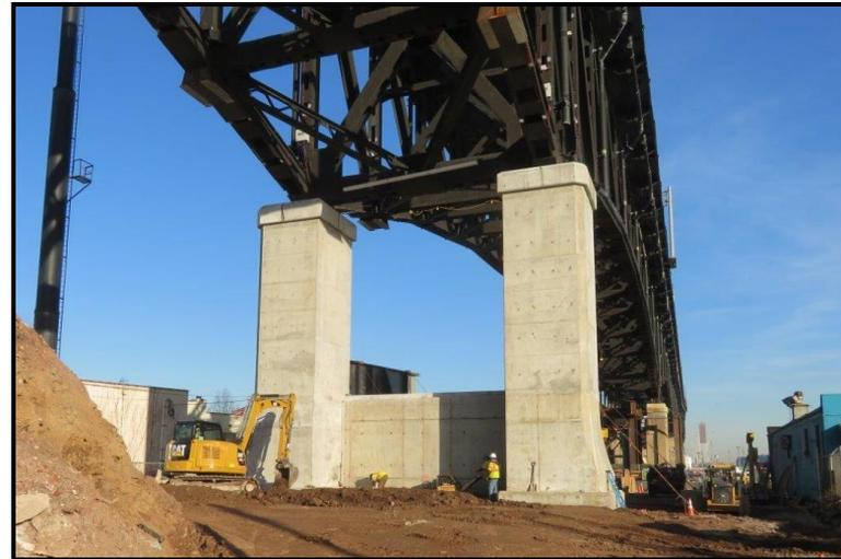
PIER 77 – SOLID PIER ELEVATION
