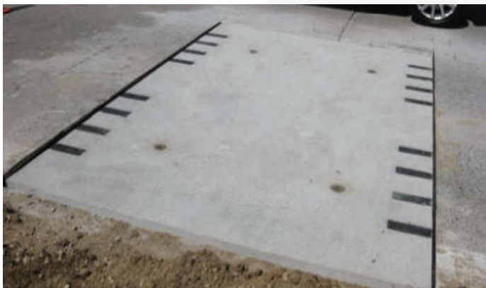
Partial Dowel Bar Retrofit 1
