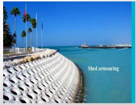
Example of a seawall similar to SEAHIVE concept. The students results found a hexagonal shape for the SEAHIVE Seawall was most effective at dissipating wave energy
