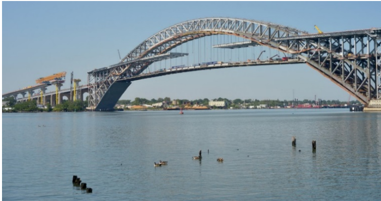
Figure 4: Bayonne Bridge Navigational Clearance Project (Source: SLLive.com)
