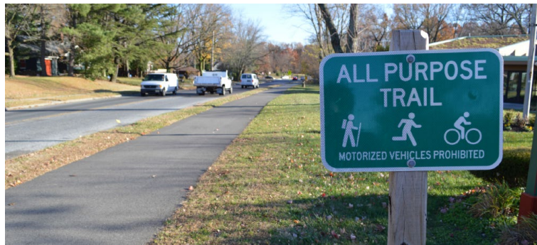
Figure 7: All Purpose Trail in Cherry Hill (Source: New Jersey Bicycle and Pedestrian Resource Center)
