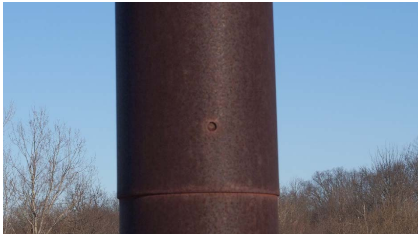
Figure 5. UAS Photograph of Potential Defect Source: NJDOT Aeronautics, 2016.
