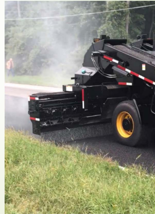
Aggregate Spreading
