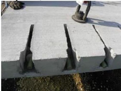
**Figure 12: Illinois Tollway modification to SHRP narrow-mouth system (from Tayabji and Brink, 2015).**
