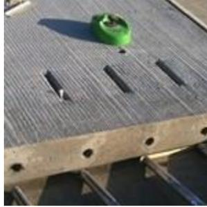
**Figure 14: Rapid Roadways Barra Glide dowel system (from [www.rapidroadway.com/Gallery](http://www.rapidroadway.com/Gallery)).**
