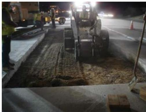
**Figure 8: A skid-steer mounted milling head used to trim a cement treated base (NCPA, 2017)**
