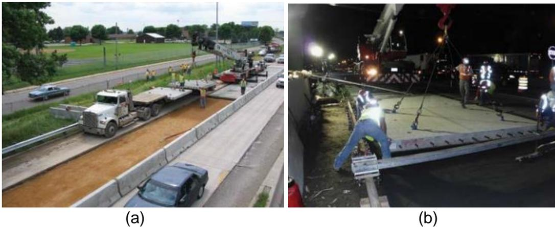
**Figure 2: (a) Single lane repair using an existing lane and the shoulder, and (b) single lane closure and placement of slabs using crane (SHRP-2, 2015)**
