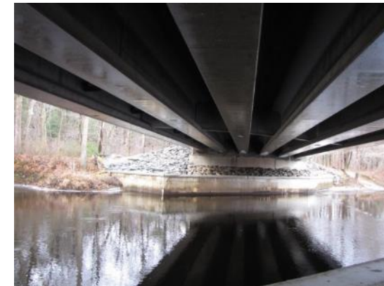
Bridge B-23-005-M-18-002, Bridgewater, MA
