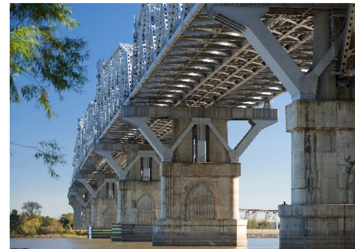
Huey P. Long Bridge in Jefferson Parish, Louisiana
