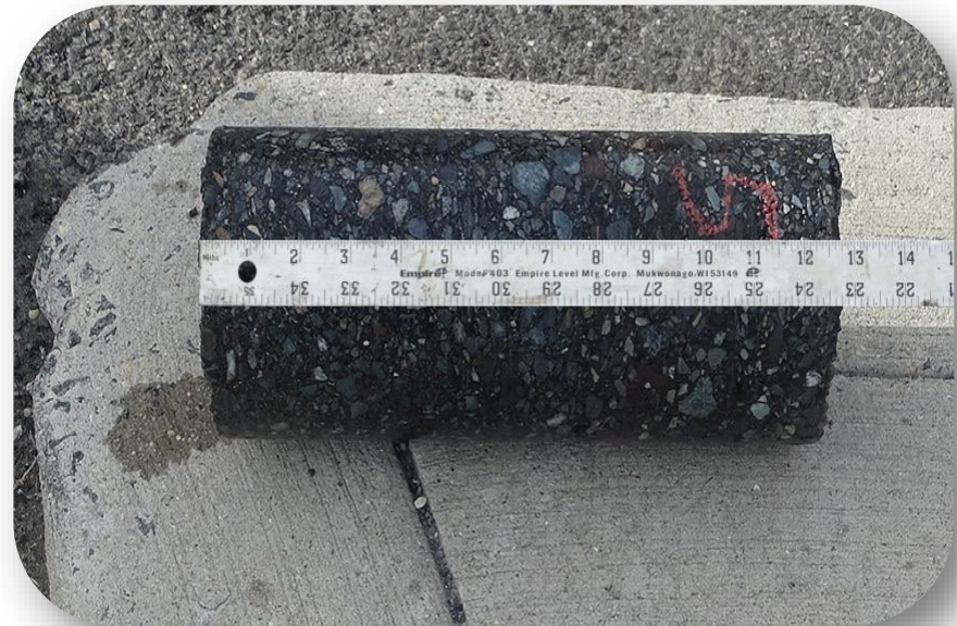
Core 5 (No HMA Stripping)
