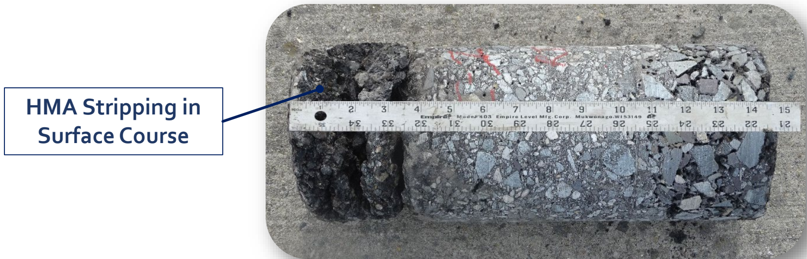
Core 1 (Failed area)
