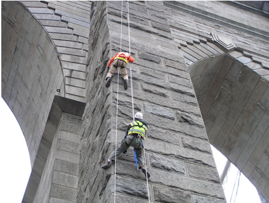
Workers rappel down the side of the Brooklyn Bridge to install highly sensitive accelerometers to measure vibrations
