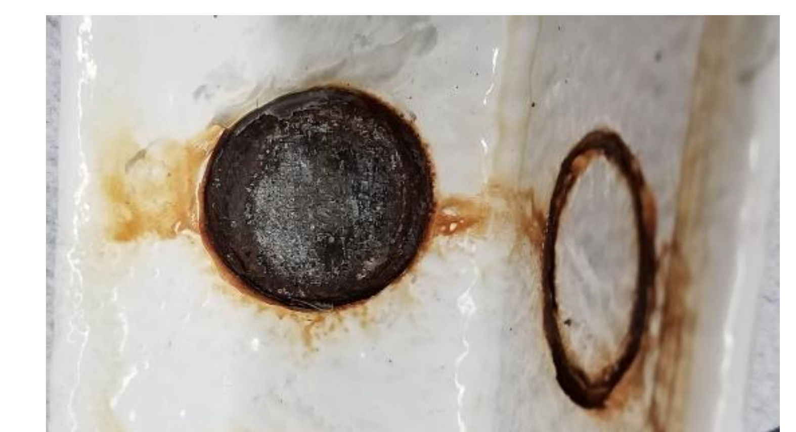
Fig.8 Enlarged view: Corrosion progresses from perimeter towards center
