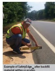
Example of SafetyEdge SM after backfill material settles or erodes.
