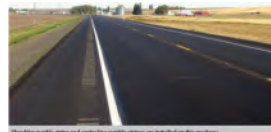
Example of center line rumble strips and center line rumble stripes installed on this roadway.
