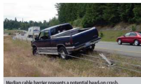
Median cable barrier prevents a potential head-on crash.
