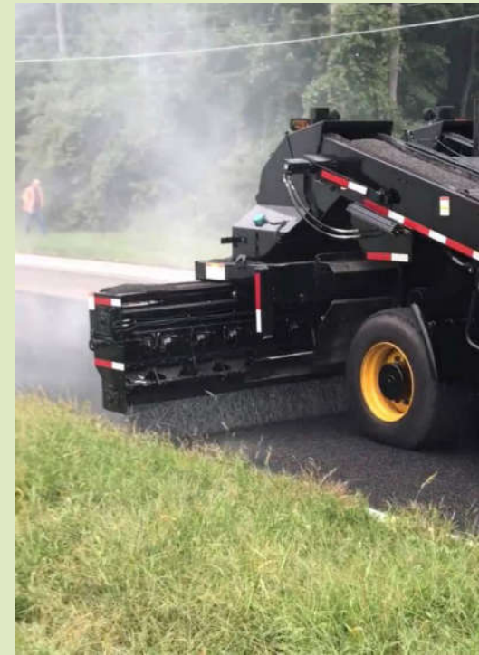
Aggregate Spreading
