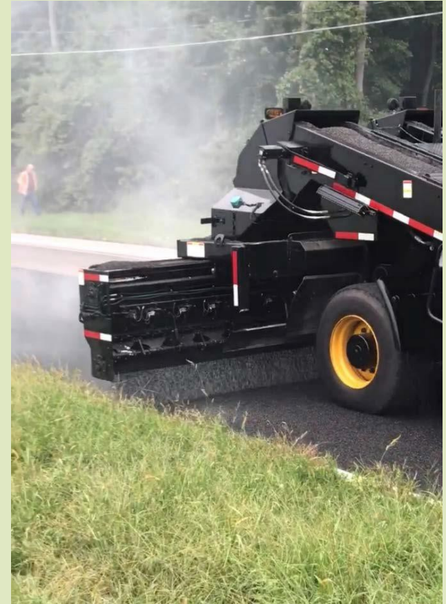
Aggregate Spreading
