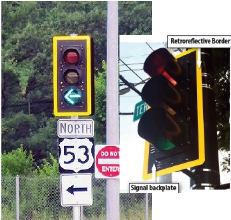
Example of a signal backplate framed with a retroreflective border.
