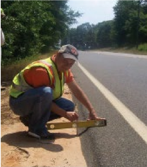
Example of SafetyEdge SM after backfill material settles or erodes.
