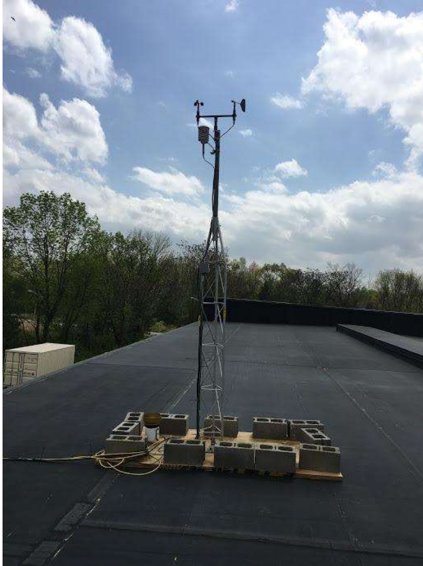
Figure 37. Rooftop weather station
