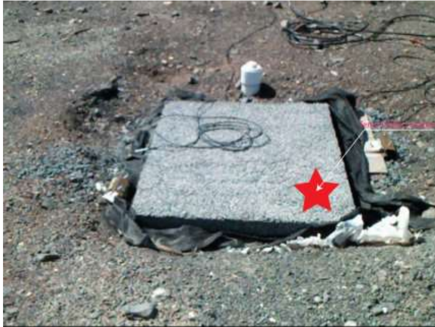
Figure 39. In-Slab temperature probe location
