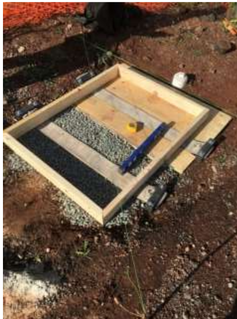
Figure 27. Placement of wooden molds before casting
