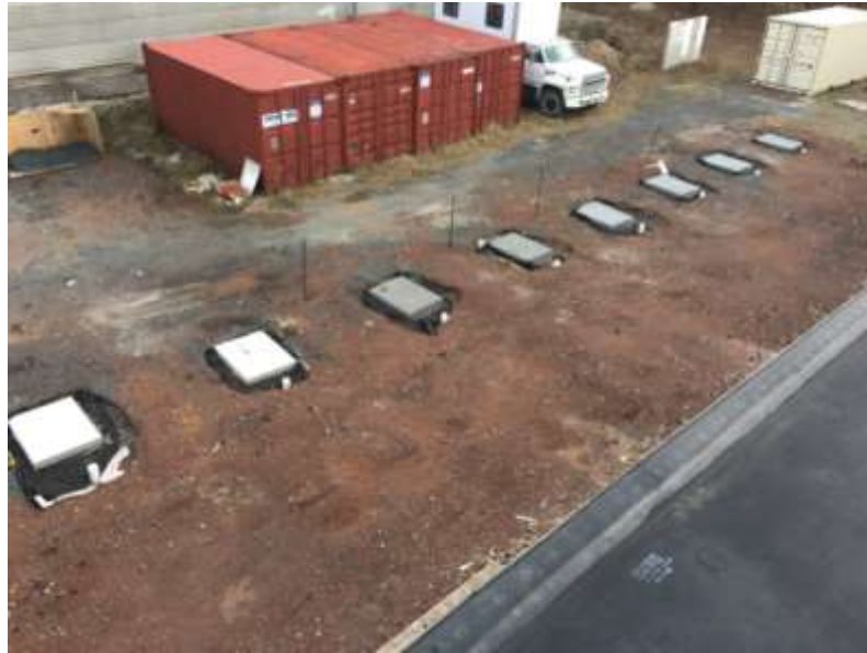
Figure 29. Completed 4 ft x 4ft x 4 in porous slab
