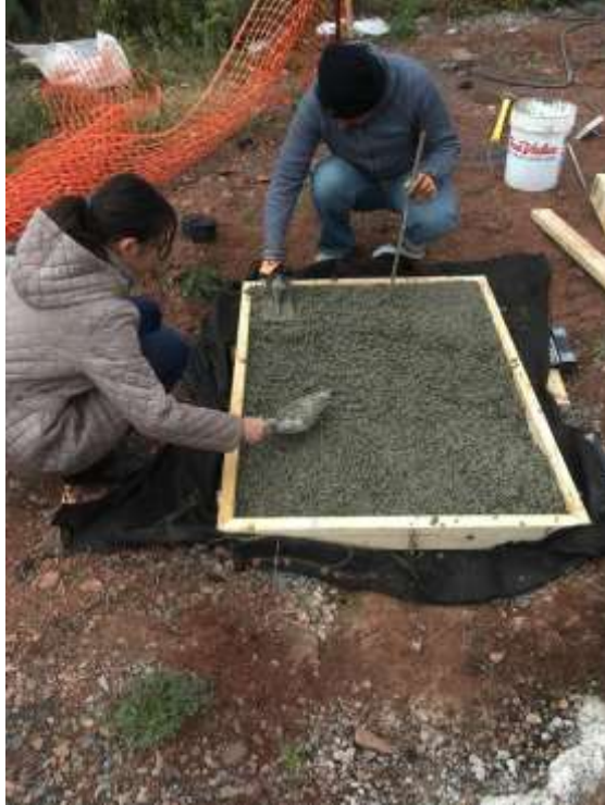
Figure 28. Rodding and finishing of a porous slab
