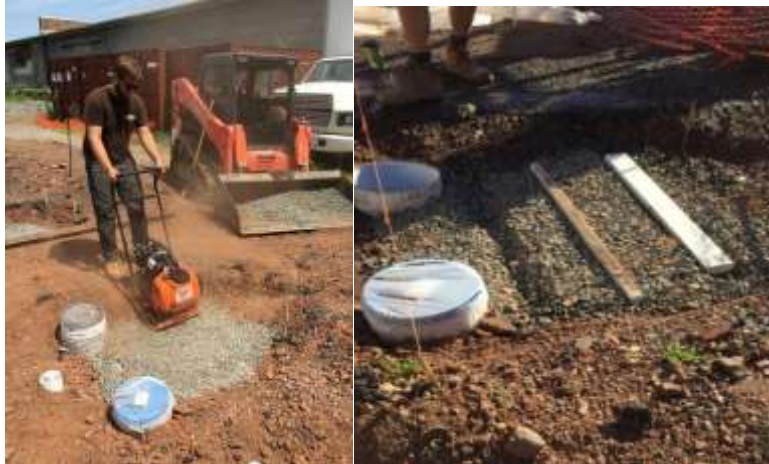
Figure 26. Preparation of subgrade and aggregate layer for field slabs
