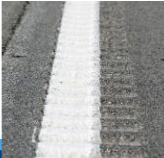
Example of an edge line rumble stripe.
