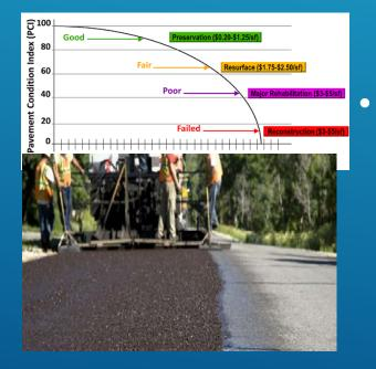
Pavement Preservation (When and Where) - developed comprehensive pavement strategy (preservation programs) that includes evaluating different pavement treatments, projecting anticipated life cycle and value information, and developing guidance to help determine appropriate treatment selection at project level
