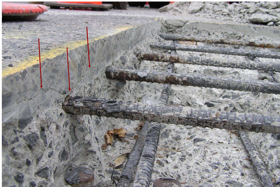
Deck Delamination
