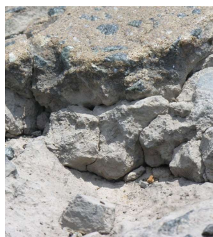
Concrete Degradation
