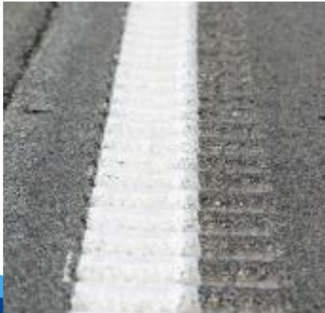
Example of an edge line rumble stripe.
