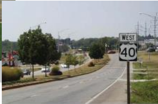
A raised median reduces conflict points along this roadway.
