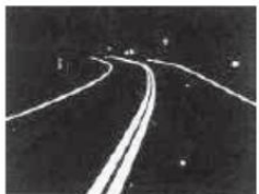
Roadway with glass beads vs. one without
